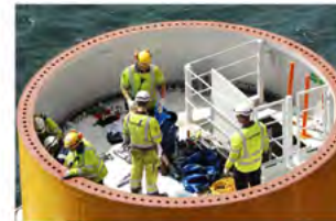
Greater Gabbard under construction
